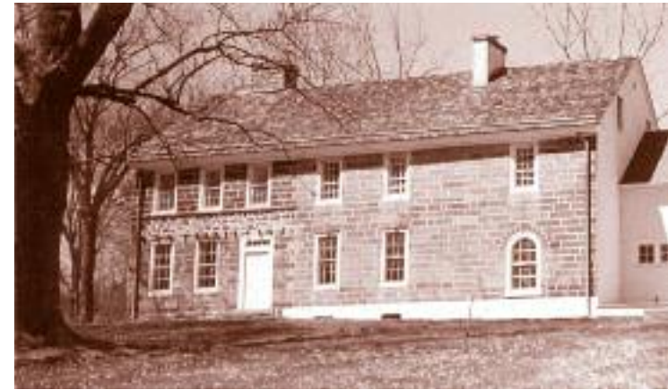
Coventry House in Chester County, Pennsylvania.
